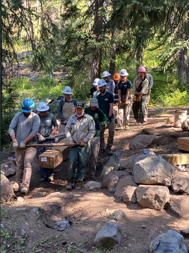
Moving a large glulam bridge stringer with the help of RMYC
