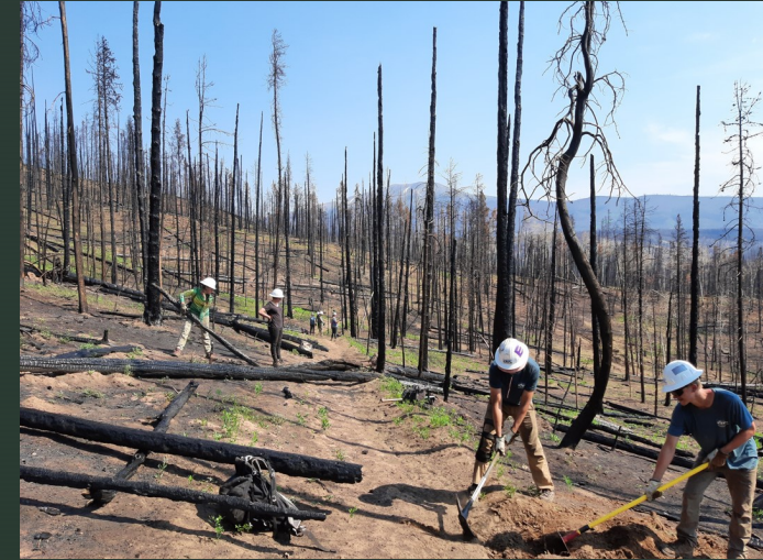
RMYC crew building drains in the East Troublesome burn scar.
