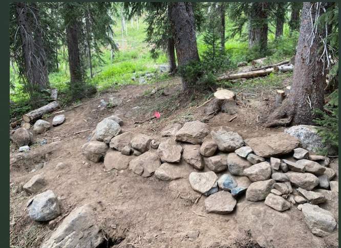
RMYC crew members working on rock bridge abutments
