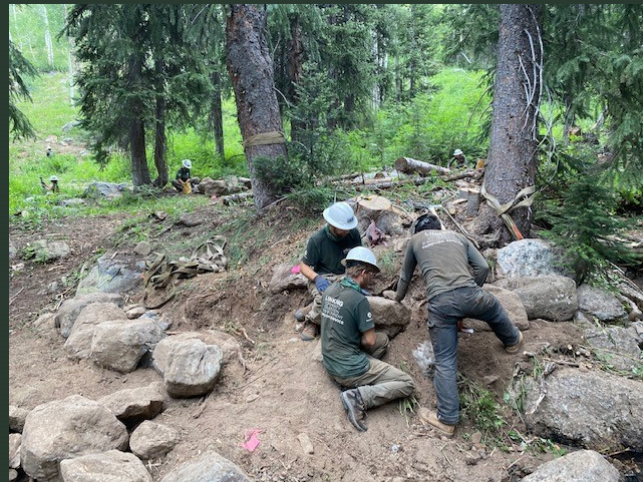
RMYC crew members working on rock bridge abutments
