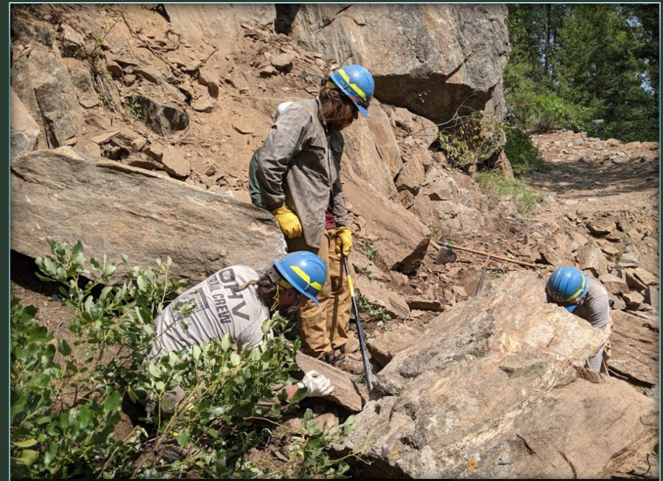
The crew utilizing rockbars and teamwork to remove large boulders off the trail
