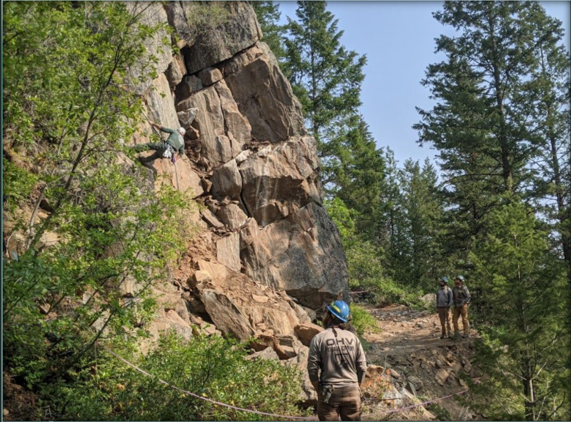
Recreation Operations Manager Steve McCone rappelling off the cliff face to remove remaining loose boulders from rock wall
